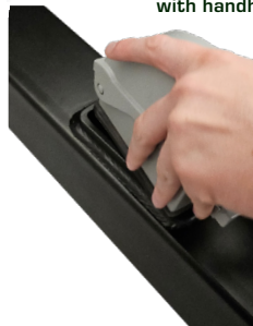
FIGURE 3 ROTATE assembly so the cover is square with handhole frame.
